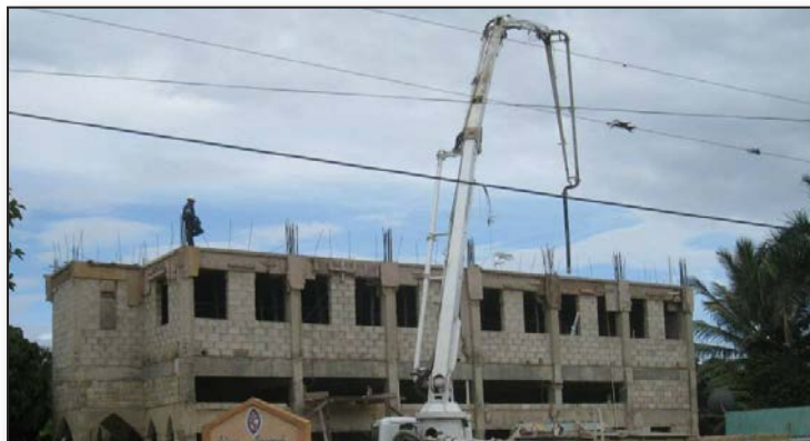
November 2013: Concrete is poured for the roof of the second floor.
