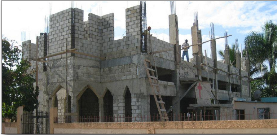
April 2013: work begins on the second floor.
