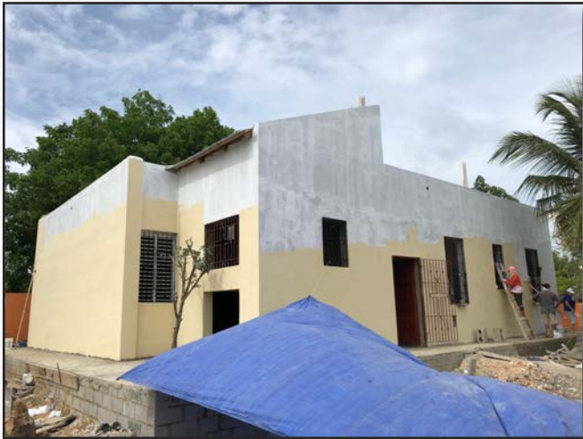
Painting the outside of the building. Pintando el exterior del edificio.
