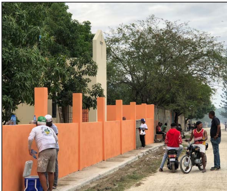
Painting the exterior wall. Pintar la pared exterior.
